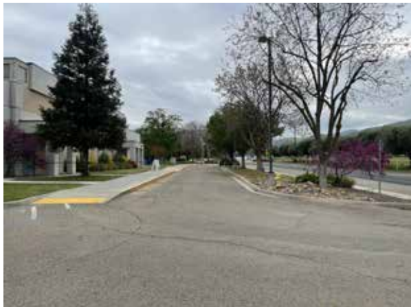
Patch and seal parking lot
