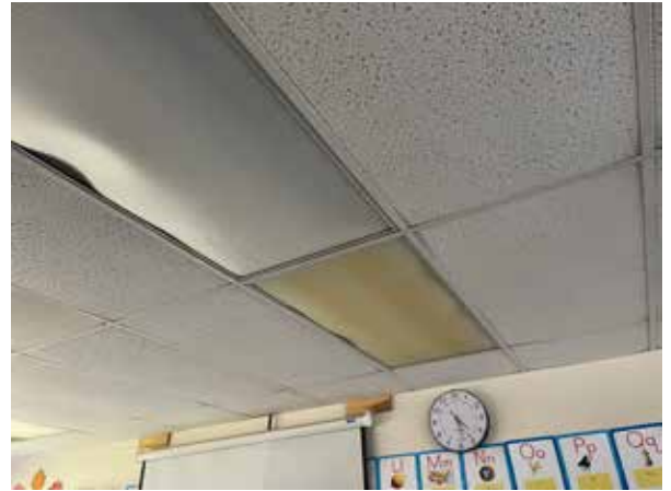
Upgrade lighting to LED
